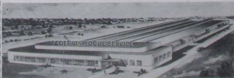
Our New Home—600 W. Chicago Street
