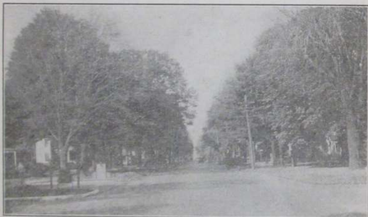
VIEW ON WEST CHICAGO ST.
