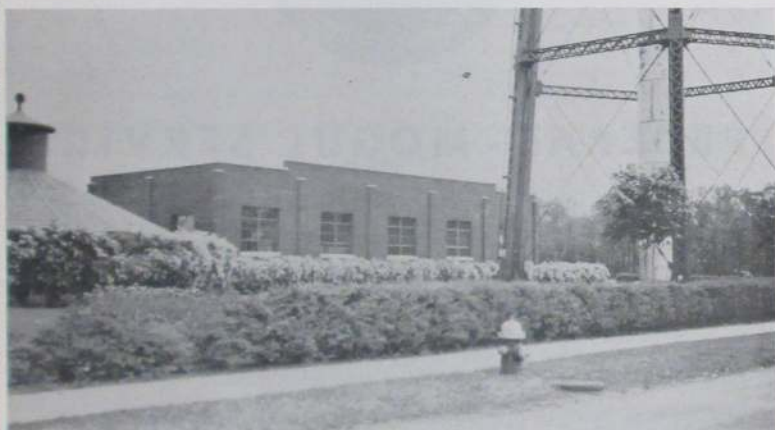
Street Scene In Front Of Water And Electric Plant
