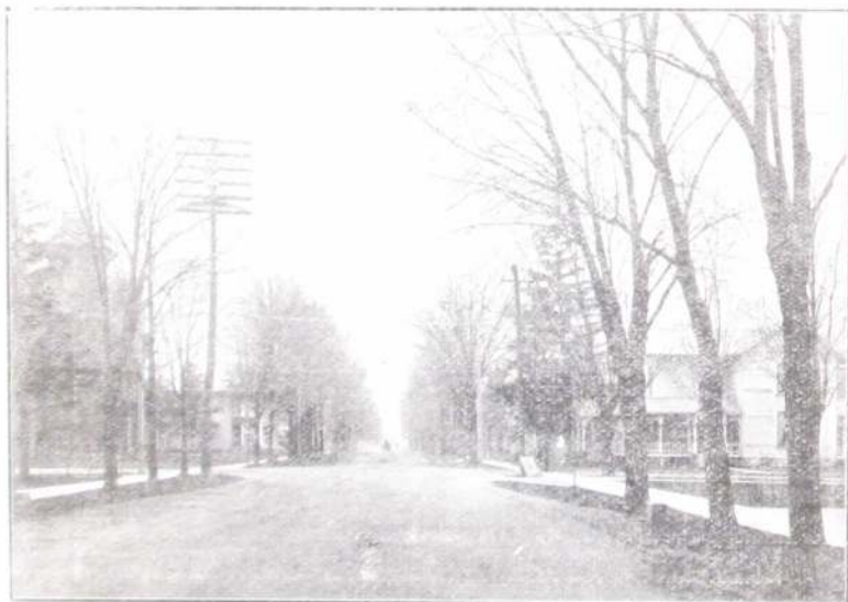
DIVISION STREET LOOKING SOUTH FROM PEARL
