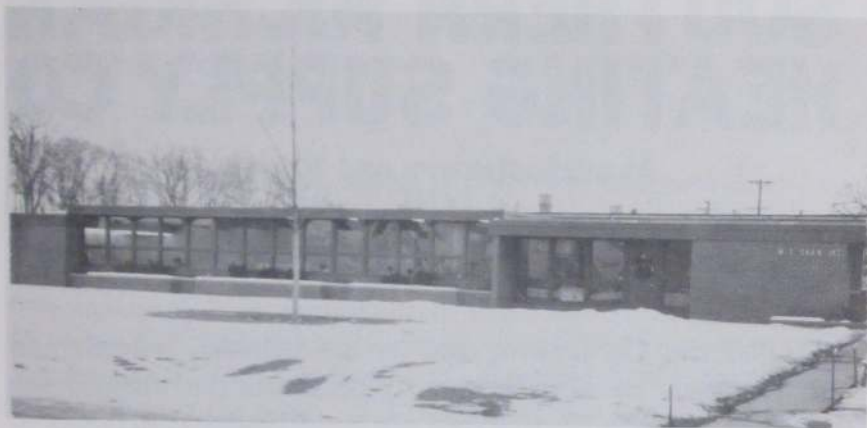
The New Offices Of M. T. Shaw, Inc., Completed In June 1960
