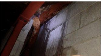
3<sup>rd</sup> floor leak, west side of 1979 portion of building It's clear that some work was done from the ground, but this is the best view we have. Chenoweth worker said flashing had been
