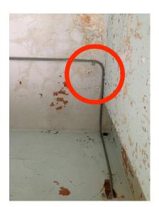
New active leak (red) above old main entrance in local history room Cause of this leak was determined by Chenoweth workers to be a piece of detached flashing.
